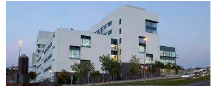
Hospital Atthaia Manresa
